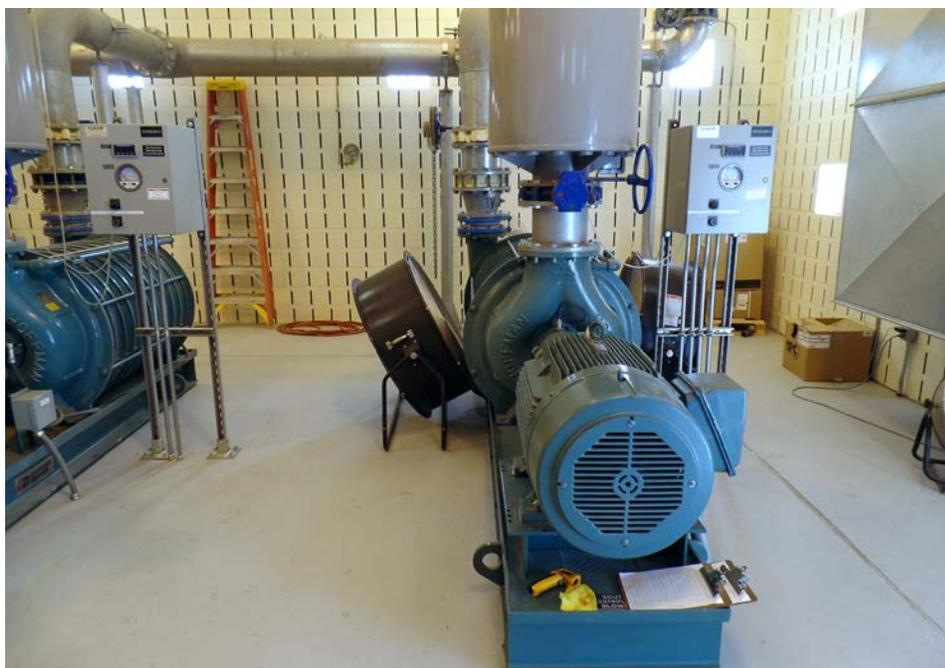
New Aerzen Delta Hybrid unit installed in "slot" previously occupied by a similar blower, shown in foreground
