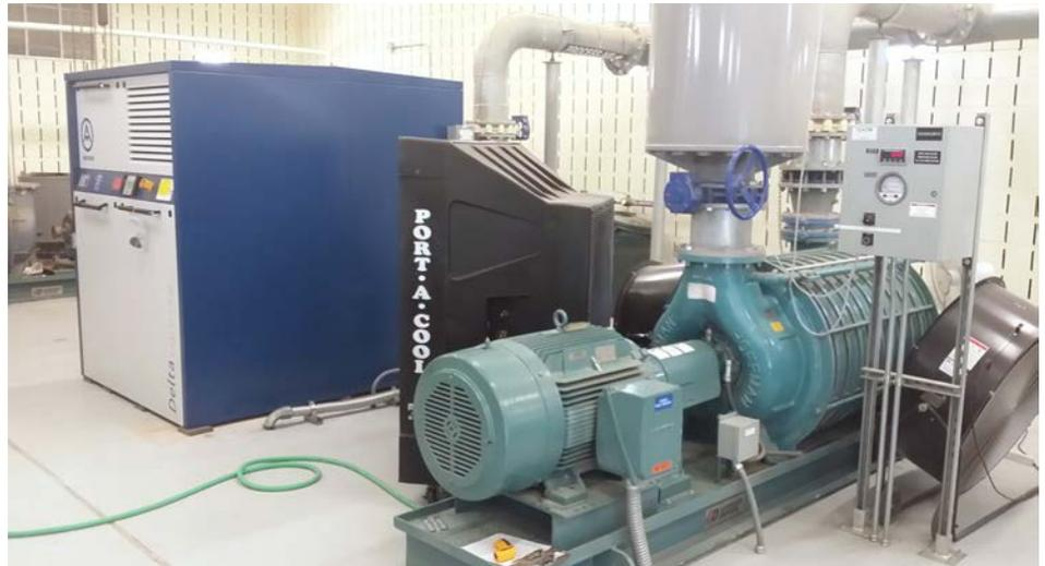
New Aerzen Delta Hybrid unit installed in "slot" previously occupied by a similar blower, shown in foreground
