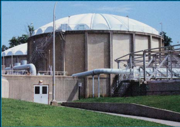
Williamsburg WWTP Hampton Roads Sanitation District Williamsburg, Virginia
