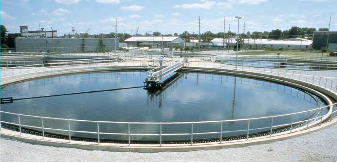
Four 110-foot diameter tanks in this wastewater treatment plant operate at an average raw flow of 400 GPD per square foot of overflow. Effluent BOD ranges from 4 to 6 ppm.
