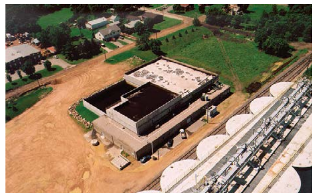
OMNIFLO® SBR installed at Rahr Malting
