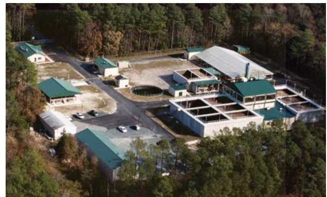
Fruitland, Maryland Wastewater Treatment Plant
