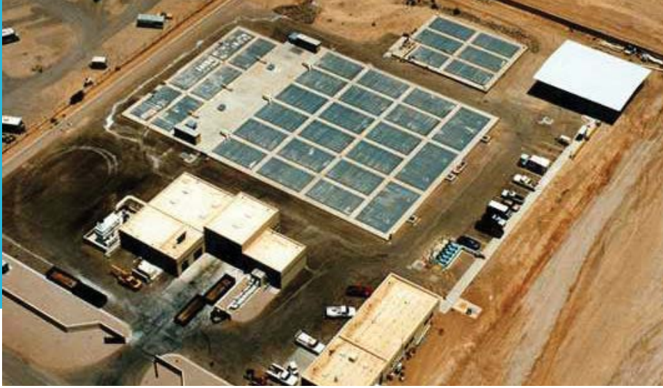
The 2.4 MGD Pima Utility Wastewater Treatment Plant meets Title 22 effluent quality standards.
