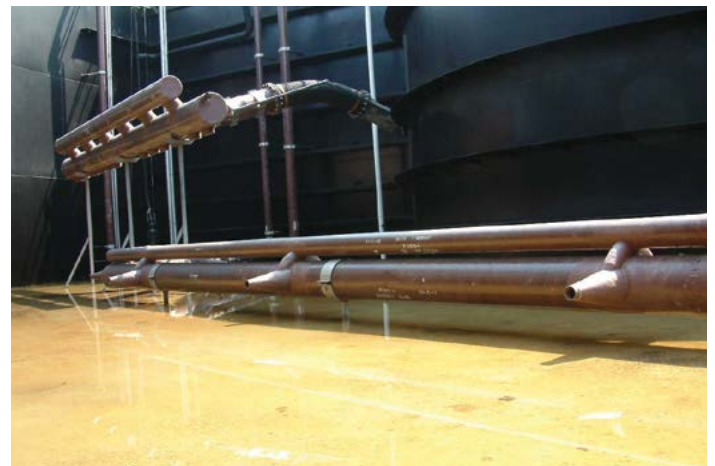
VARI-CANT® Jet Aeration System and Floating Solids Excluding Decanter from Evoqua installed in OMNIPAC® Field-Erected SBR system.
