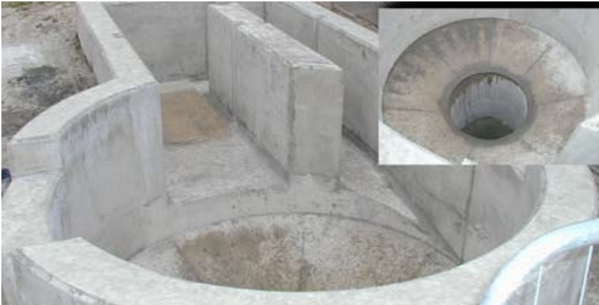
Civil construction and installation.
