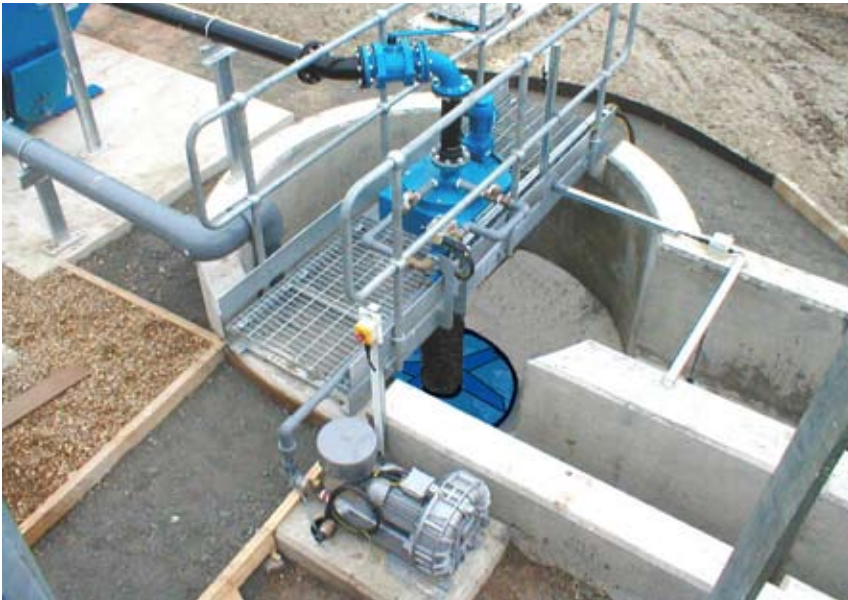
The completed JetAir installation.
