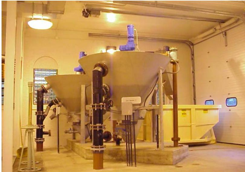
La Crosse knew that the organics were the problem. The weight and quantity of the grit was compounded by its accompanying organics. By putting a process in place to wash the grit, the organics would be removed and its cost of disposal reduced by weight and hazardous materials rates. If organics could be subjected to removal and further treatment, both the grit and the resulting organic material could be turned into useful by-products and more easily and economically removed from the plant.
