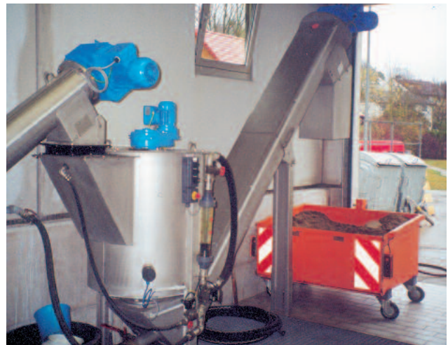
Grit Washer RoSF 4/t fed with classified grit from a ROTAMAT® Complete Plant
