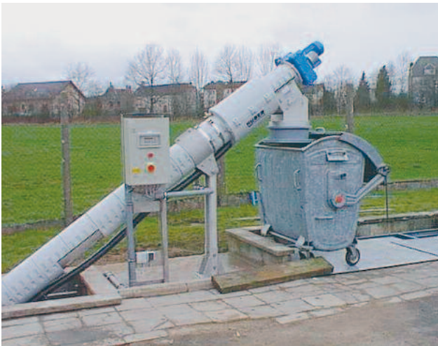
Outdoor installation of a ROTAMAT® Ro 1 Cylindrical Bar Screen with frost-protection and bagger
