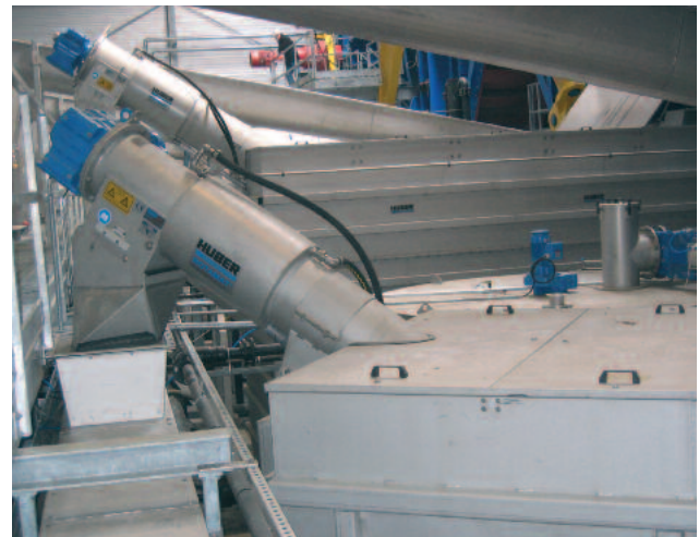
... available with basket diameters from 2 to 8 ft (0.6 to 2.4 m)
