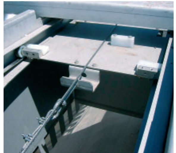
Automatic grease removal by means of a paddle system
