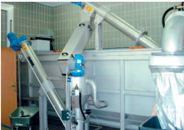
Classifying screw with subsequent HUBER Grit Washer RoSF 4/tC
