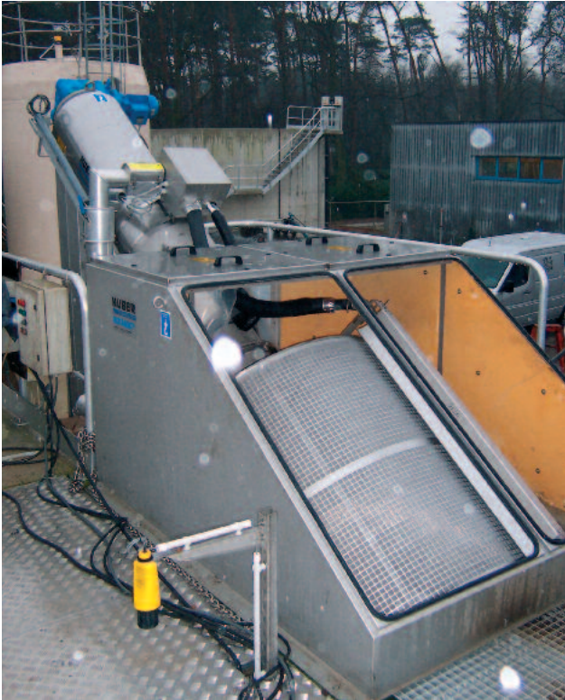
Example of an in-channel installation with protective cover.
