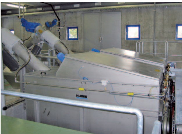
Example of an installation incorporating the use of a self contained tank and cover.
