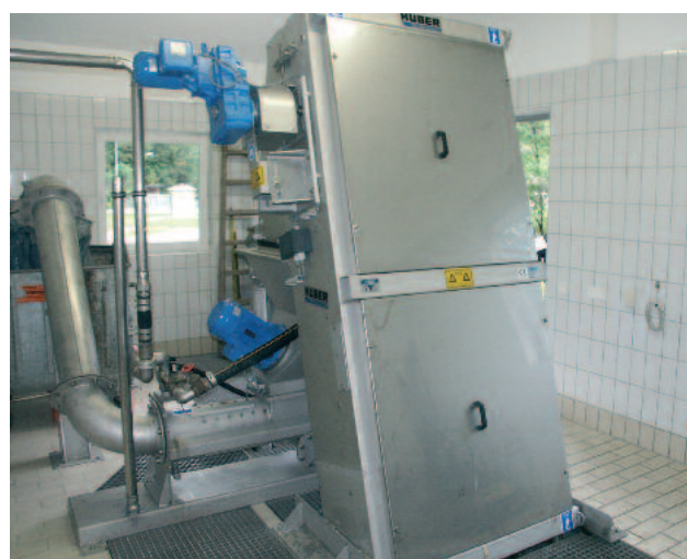
1/4 inch (6 mm) RakeMax feeding into a Super-Launder Washpress WAP/SL for perfect screenings washing and compaction
