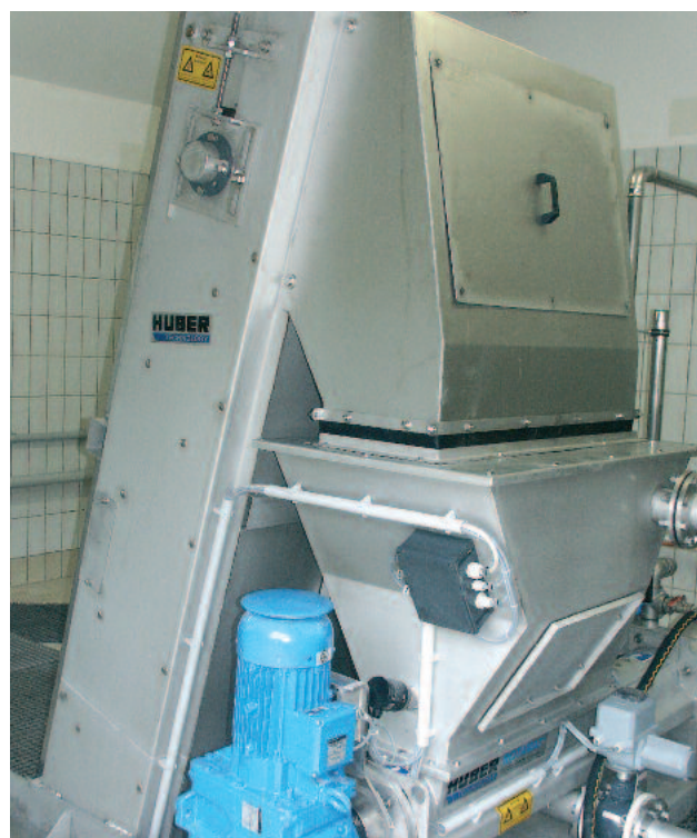
Complete enclosure for odor control; the chain tensioning system at the side of the frame is easily accessible
