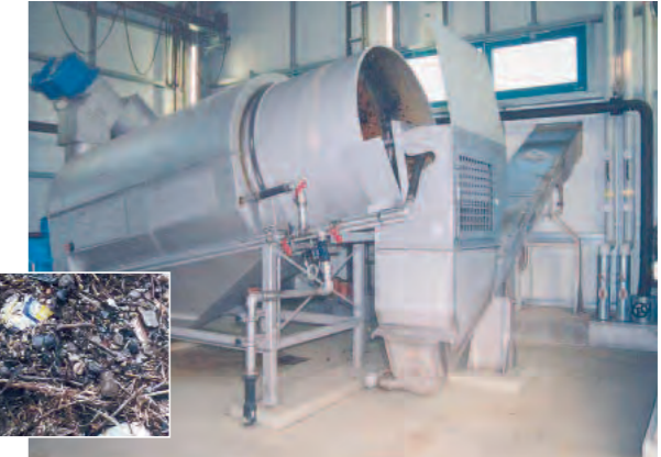
ROTAMAT® Wash Drum for washout and separation of all coarse material > 3/8" (10 mm)
