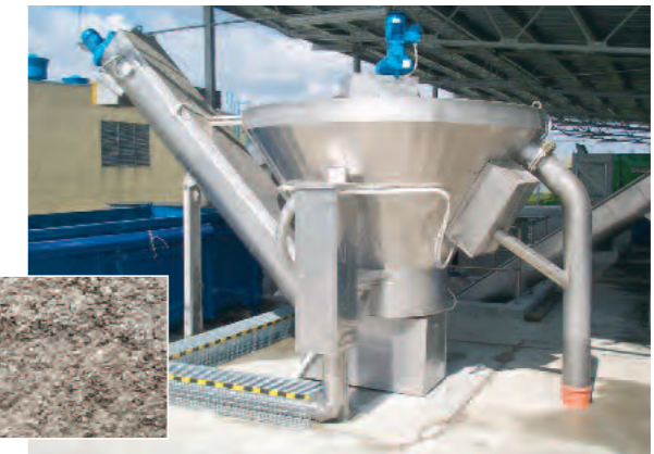
Washed grit from COANDA Grit Washer with < 3% loss on ignition, particle size up to 3/8" (10 mm), DR > 90%
