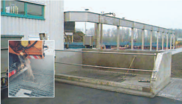
Acceptance tank with bar grate and integrated vertical dosing screw
