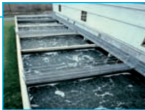
Typical BIOFOR® installation
