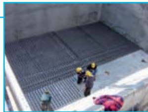
Nozzle installation in filter
