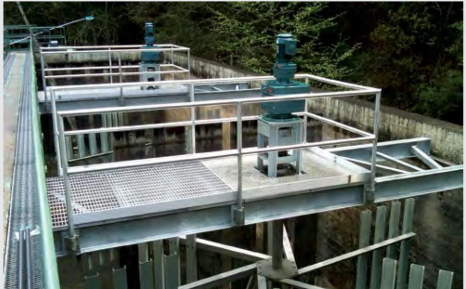
*Ashland, OR Mega-FLOC (VPWF) Installation with Bridge Assembly and Integral VFD (MOVIMOT®)*
