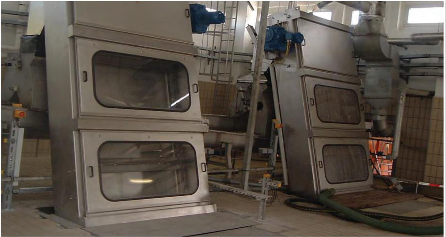
The WasteTech Multi-Rake Bar Screen combines fine or coarse screening with high solids capture rates. Its robust construction and overload feature ensure reliable operation.
