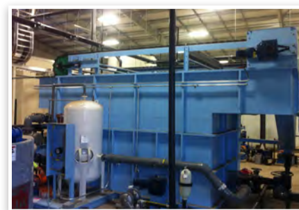
DAF Unit Using Conventional Recycle System.
