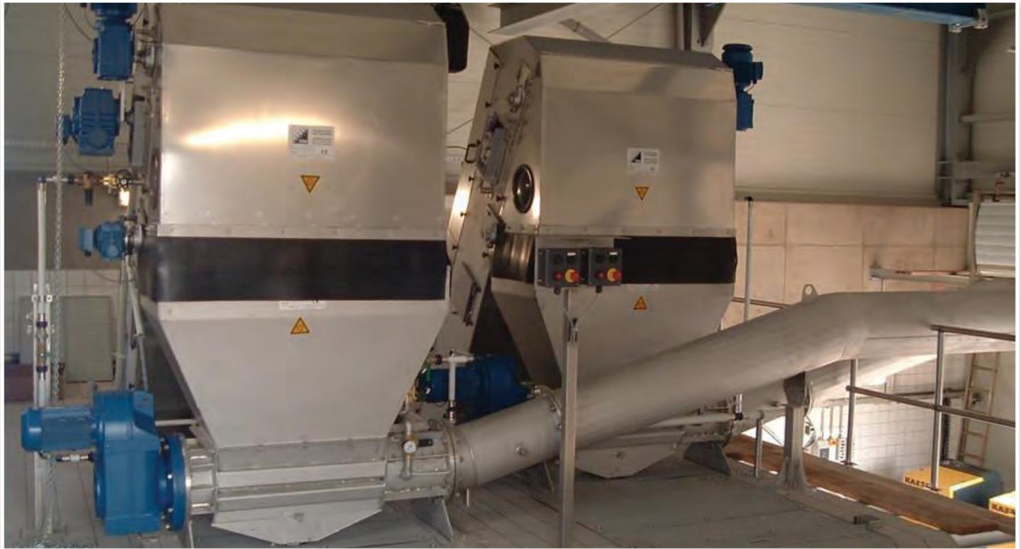
The FSM Washer Compactor reduces the weight and volume of screenings while washing out more than 95% of fecal matter, combining high performance with low operating costs.
