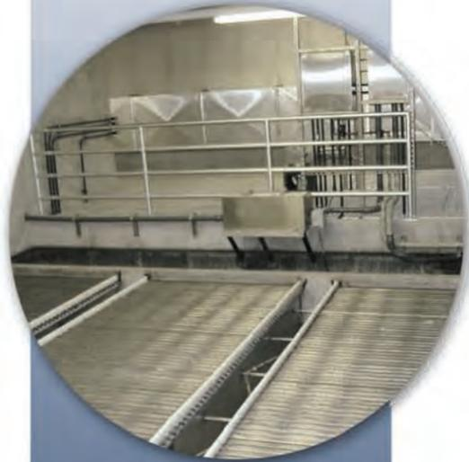
BROOMFIELD WATER TREATMENT PLANT, COLORADO—THIS CITY NEEDED TO EXPAND PLANT OPERATIONS BY 100% ON A PROPERTY THAT WAS ALMOST FULLY UTILIZED, SO ANY MODIFICATIONS HAD TO BE VERY COMPACT. INCLINED PLATE SETTLERS WERE INSTALLED IN THE FILTER BACKWASH RECLAIM SYSTEM IN AN UNDERGROUND VAULT, AND TODAY ARE TREATING 6,000 GALLONS PER MINUTE—WITHOUT CHEMICAL FEED.
