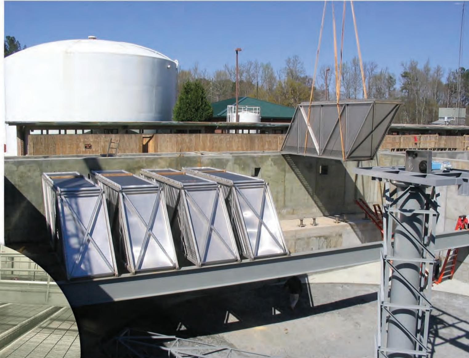
**W. J. HOOPER WATER TREATMENT FACILITY, CLAYTON COUNTY GEORGIA – THE MRI INCLINED PLATE SETTLERS ARE BEING INSTALLED IN THREE SQUARE BASINS WITH CIRCULAR CENTER DRIVE MECHANISMS. STAINLESS STEEL PLATE PACKS BY MRI WERE SELECTED FOR THEIR QUALITY, DURABILITY AND EASE OF INSTALLATION.**
