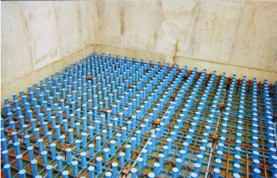
*Nozzle adapters with threaded plugs are snapped into the forms and reinforcing rods are doweled into the filter walls.*
