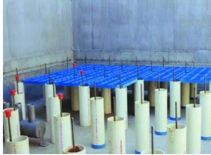
*Shims are used to adjust the height of the columns ensuring the polystyrene forms are level.*
