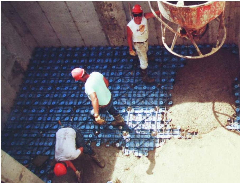
*After the concrete is poured, the resulting underdrain will withstand applied loads from above and below during filtering and backwashing operations.*
