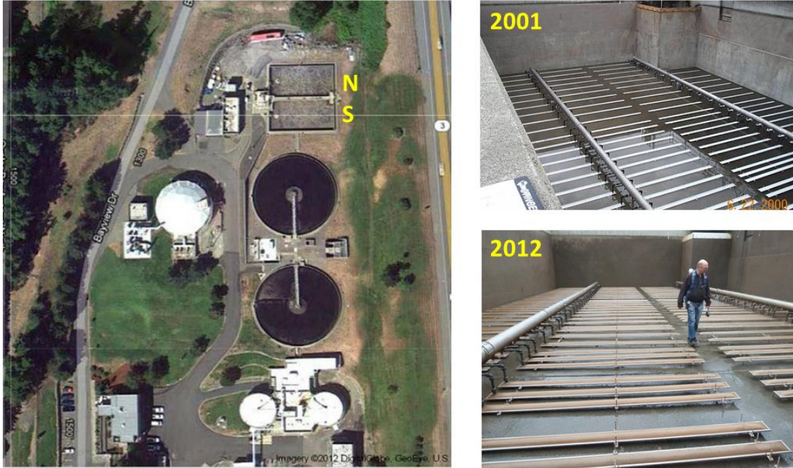
Figure 1. Bremerton Plant. Left photo shows the two basins. Top right photo shows the north basin shortly after installation and the bottom right photo shows the north basin immediately following the 2012 off gas testing.
