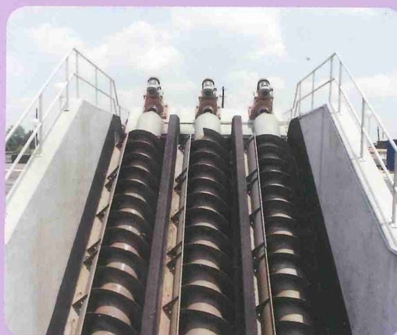
Open Flight Screw Pumps with sizes from 20" to 108" in diameter. Lift capability up to 30'.
