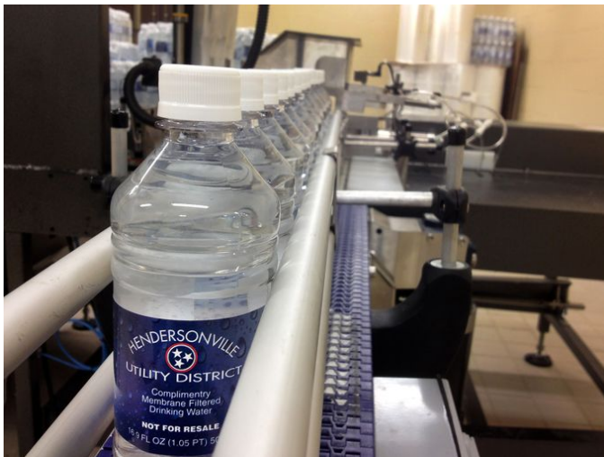
The new water treatment plant of the Hendersonville Utility District features a bottled water manufacturing line.
