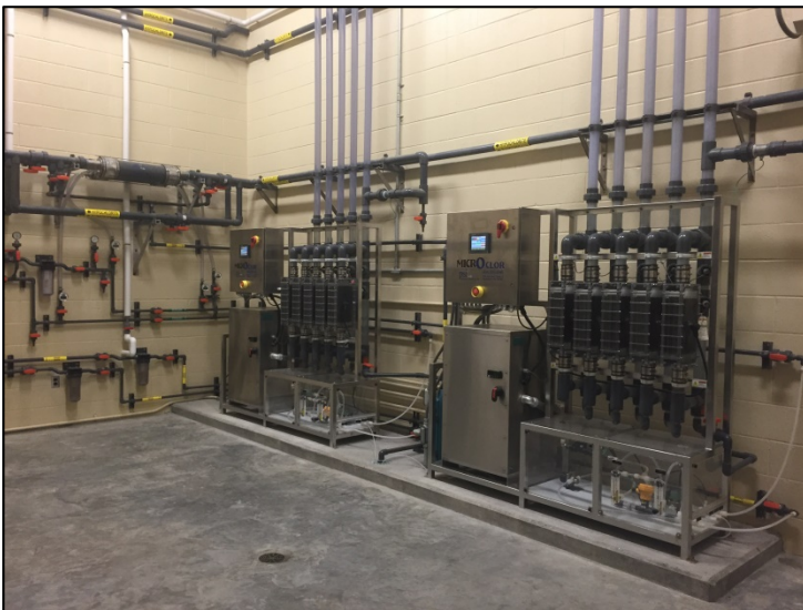
600 ppd MicroOclor™ On-Site Hypochlorite System
