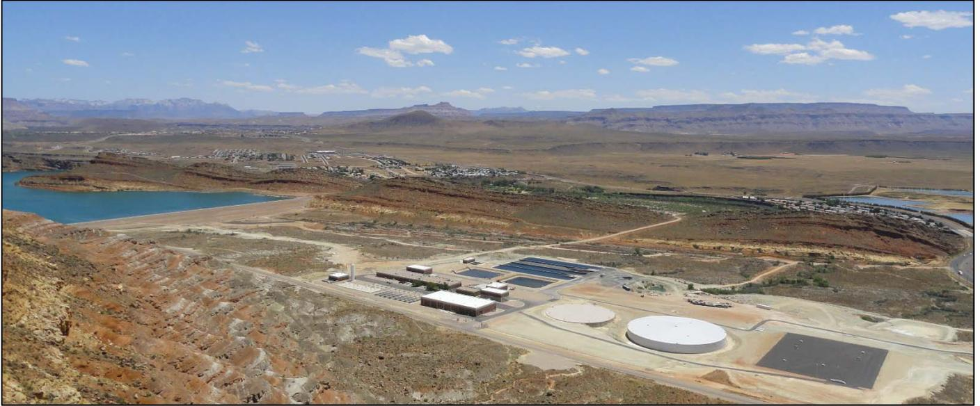
**Originally built to treat 10 million gallons per day (MGD), the Quail Creek Water Treatment Plant in Washington County, Utah, now has an operational capacity of 60 MGD and a design capacity of 80 MGD. Quail Creek Reservoir is shown to the left.**
