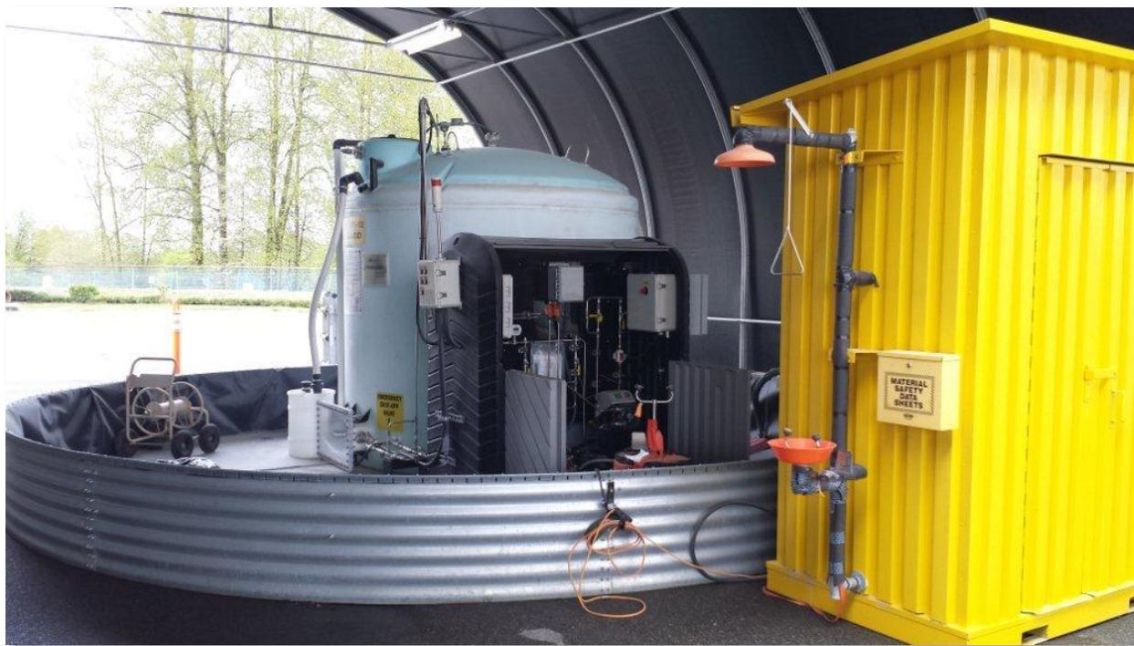
**Figure 2: Peracetic Acid System Installation at Northwest Langley Wastewater Treatment Plant**
